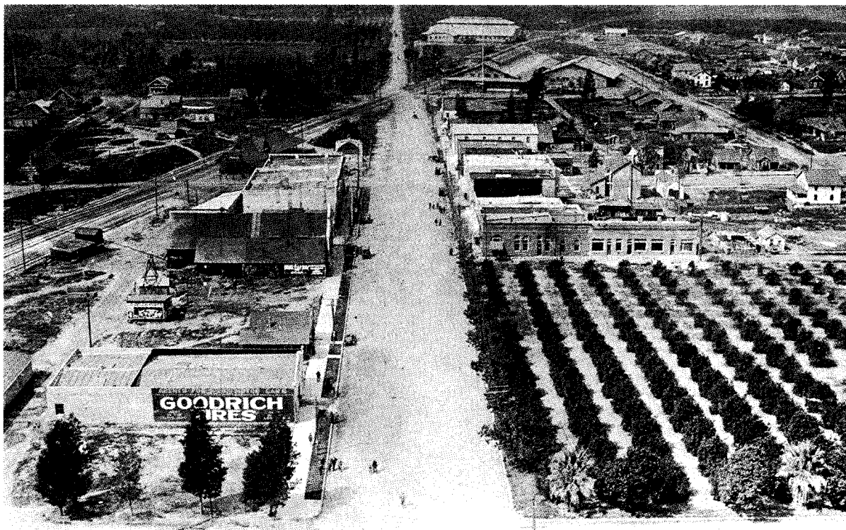
AERIAL VIEW OF BONITA AVENUE LOOKING WEST - 1914
